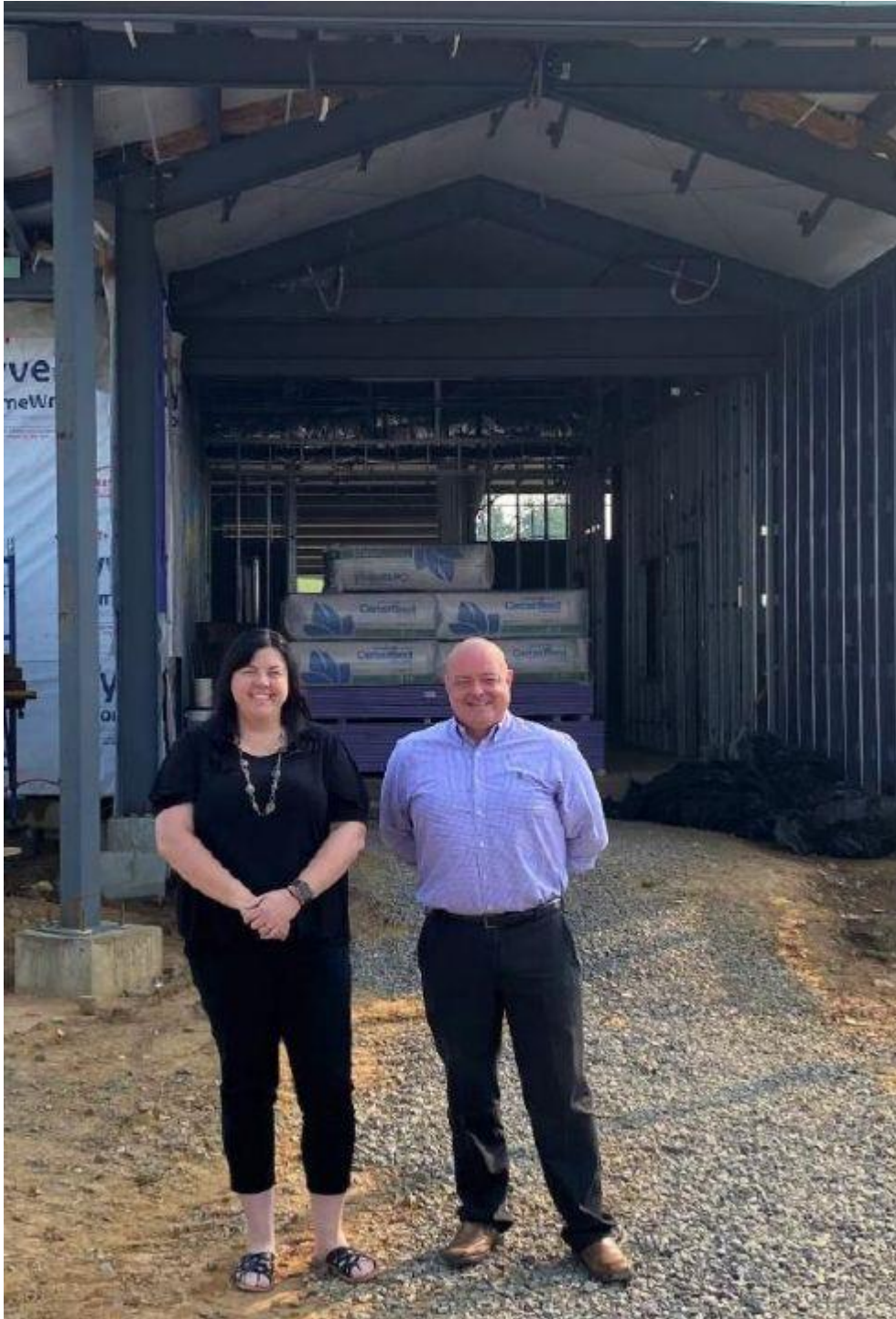
McCraw and Falls at the under-construction Aquatic Center site.
